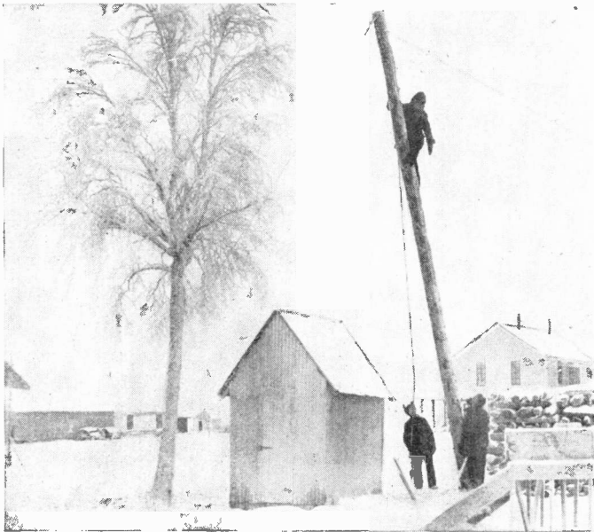
Locating a Line in Mountain Regions. Building a Line in the Dead of Winter
