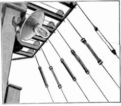
ARRANGEMENT FOR RAISING AND LOWERING ANTENNA WIRES
