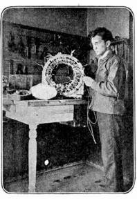
WINDING AN ARMATURE
