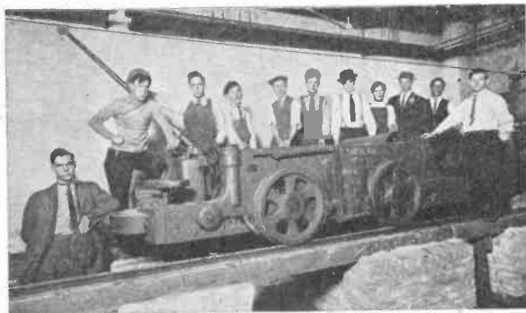
Electric Locomotive Owned by School on Which Students Are Given Practical Instruction
