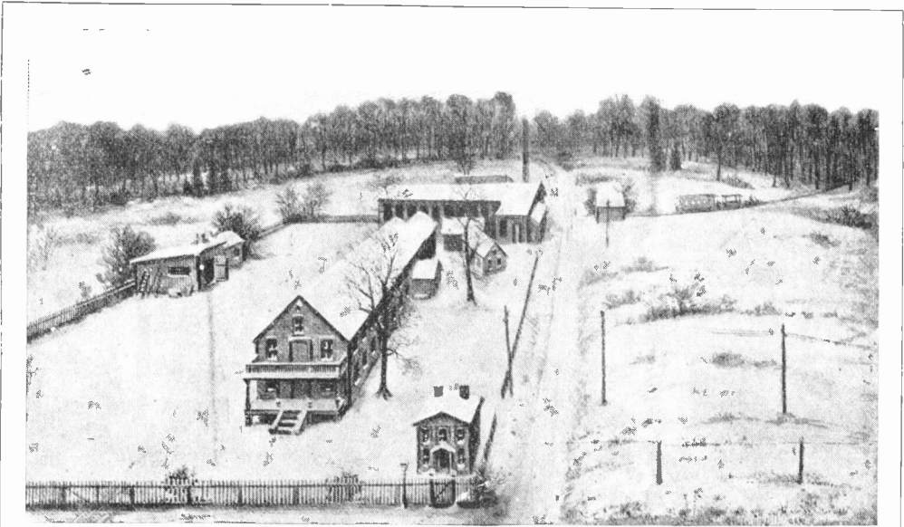
Courtesy of the Cassier Co. THE EDISON LABORATORY AT MENLO PARK IN 1879, SHOWING OUTDOOR POLE CIRCUITS ERECTED FOR THE FIRST PUBLIC EXHIBITION OF INCANDESCENT LAMPS
