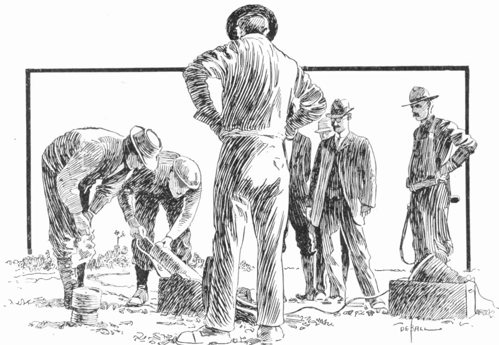
GETTING READY TO FIRE THE LINE ACROSS THE RIVER
