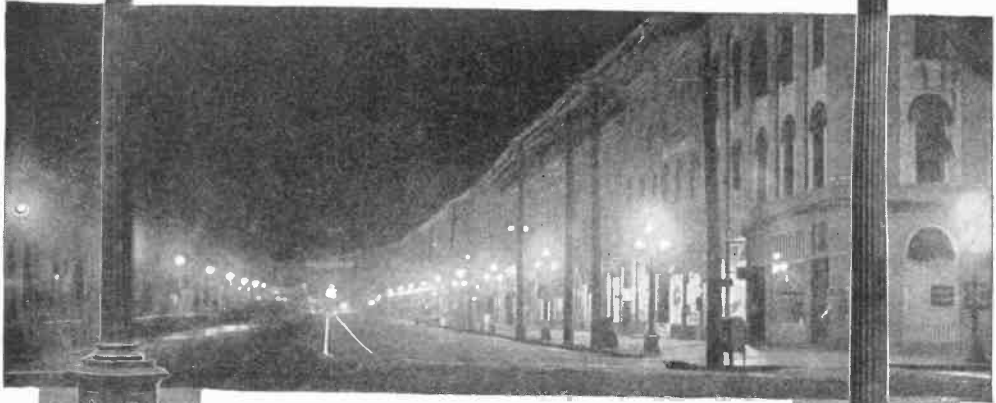
STREET SCENE IN WARREN, OHIO, SHOWING ALSO TYPES OF ORNAMENTAL FIXTURES
