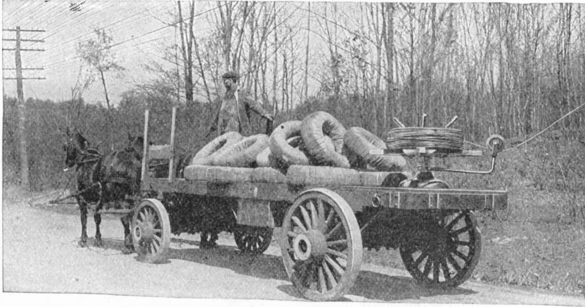
STRINGING WIRE FROM A SPECIALLY CONSTRUCTED BLADE
