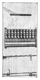
FIRST EXCHANGE SWITCH BOARD WITH TWENTY CIRCUITS EQUIPPED IN 1878
