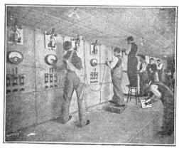
GENERAL VIEW OF MAIN SWITCH BOARD SHGW-ING STUDENTS EQUIPPING BOARD FOR HANDLING ALTERNATING AND DIRECT CURRENT
