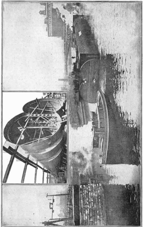
GIANT TUBES FOR ELECTRIC RAILWAY TUNNELS UNDER THE CHICAGO RIVER, AND HOW THEY WERE FLQATED INTO POSITION
