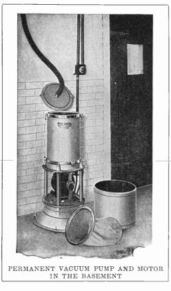
A little piping will be necessary, but not nearly so elaborate as for the heating and plumbing which are now recognized necessities. One way of acquiring this most desirable adjunct to a modern home is by the use of what is known as the Keller-Duplex system, which is shown in the illustrations.
