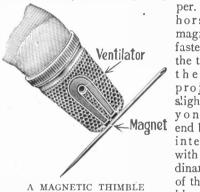
per. A little horseshoe magnet is fastened to the thimble. the ends projecting slightly be-yond the end but not inter fering with the ordinary use of the thimble. This
