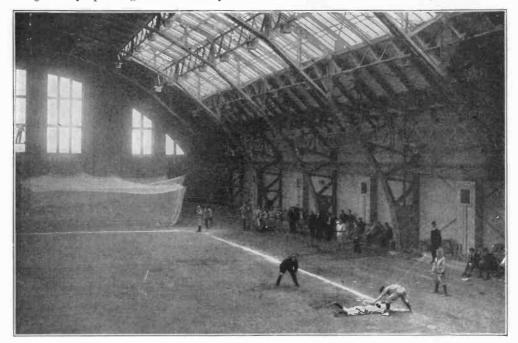
BASE BALL CAGE AND RUNNING TRACK ILLUMINATED BY BOTH DIRECT AND INDI-RECT SYSTEMS
