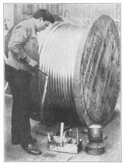
FIG. 7. SEALING UP THE END OF A TELEPHONE CABLE
