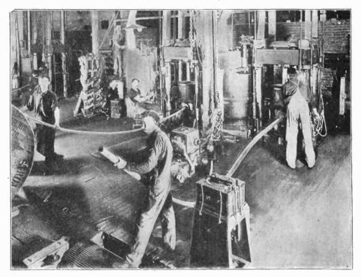
FIG. 4. FINISHED CABLE COMING OUT OF THE LEAD PRESSES. THE LEAD JACKET IS SMOOTH AND CYLINDRICAL, WITHOUT A SEAM
