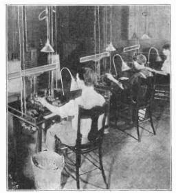
FIG. 5. TESTING NEW-MADE CABLE-IN THE LABORATORY
