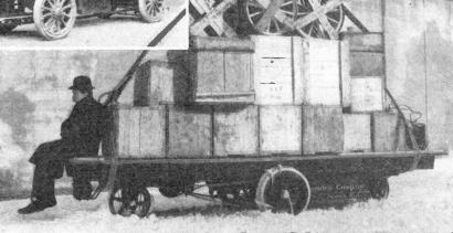
TRUCK EQUIPPED WITH NEW EDISON BATTERY
