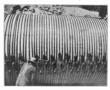
PIPE LINE OF WOOD STRENGTHENED WITH BANDS OF STEEL
