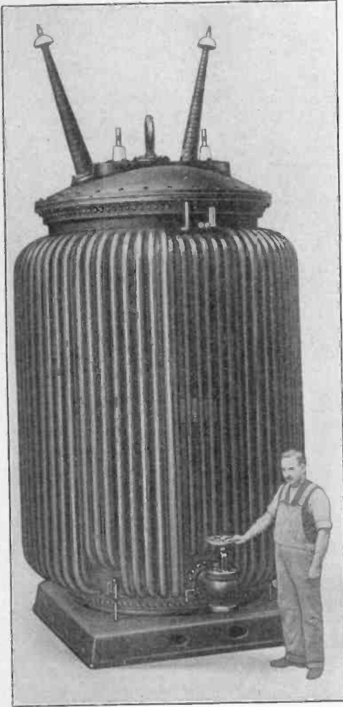
THE LARGEST SELF-COOLING TRANSFORMER
