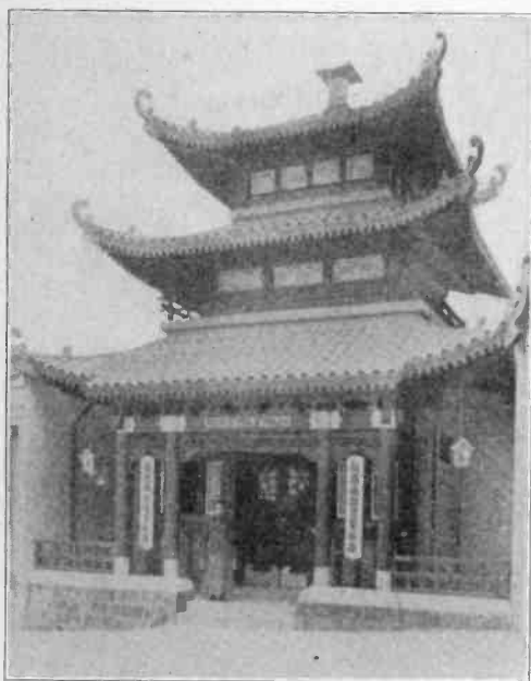
TELEPHONE EXCHANGE IN CHINATOWN
