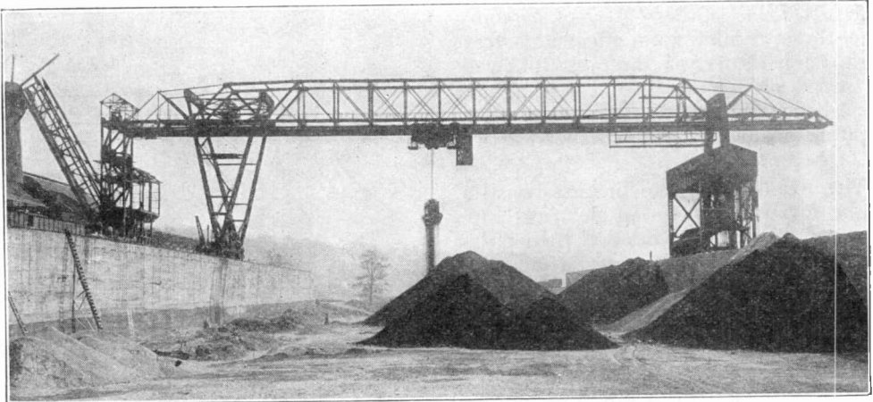
MOTOR OPERATED TRAVELING BRIDGE FOR HANDLING ORE.
