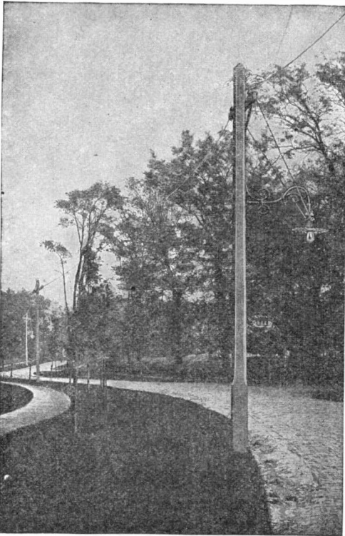
STREET LIGHTING WITH TUNGSTENS.
