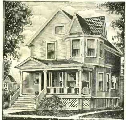
THIS IS AN EXACT PHOTOGRAPH OF OUR WONDERFUL $650 HOME. That means we will furnish you all the Lumber and Building Material needed to construct it. Write for our "Book of Plans," which gives details showing exactly which material is furnished. Mention Design "J F 5." This is only one of many other designs shown in our grand "Book of Plans."
