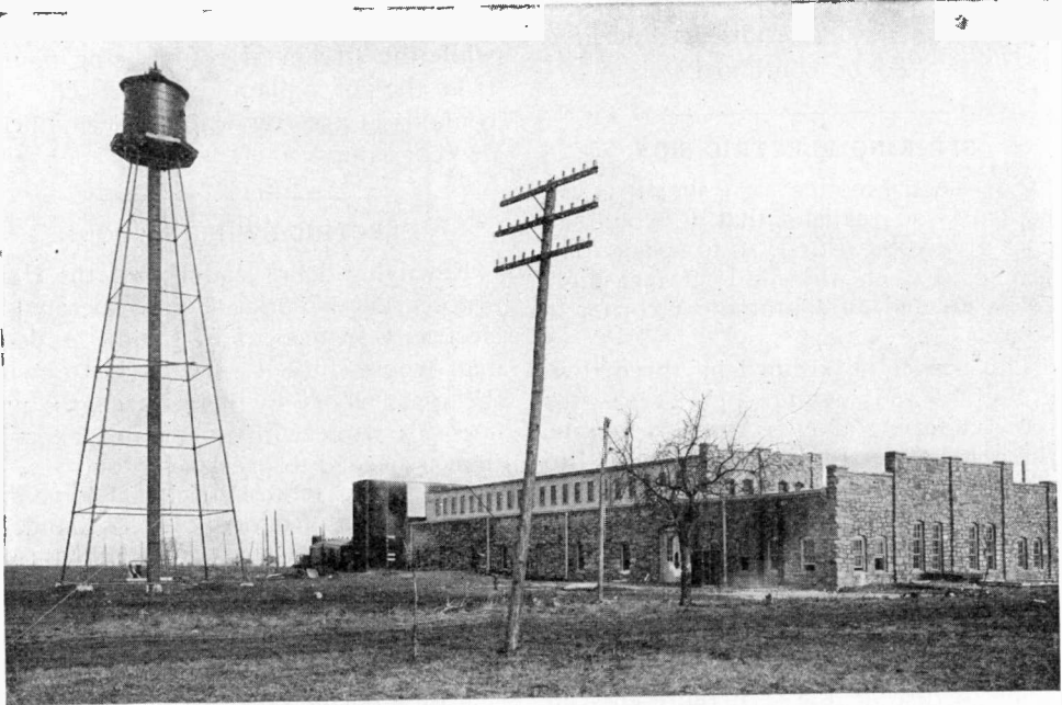
POWER HOUSE OF THE MISSOURI AND KANSAS INTERURBAN RAILWAY.
