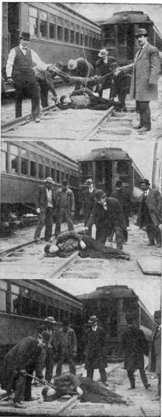
HOW TO REMOVE A VICTIM FROM CONTACT WITH A CHARGED WIRE OR THIRD RAIL.
