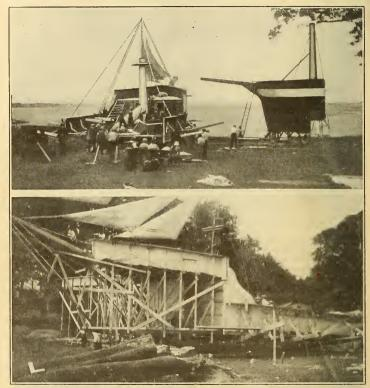
Showing Construction of Two Sailing Vessels Used in Edison's "Hard Cash". They were Built on Rockers or Cradles so They Could be Tilted Back and Forth
