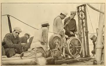
Instrument Used on United States Naval Steamship to Determine Depth of Water at a Particular Point
