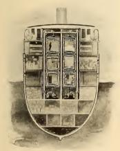
Novel Plan to Hang a Ship's Cabins in an Elevator and Control Their Action Electrically
