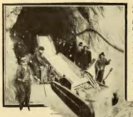
A Mucking Machine at Work in The Tunnels—Far Ahead of Hand Labor for Rapidly Removing Excavated Material from the Working Face
