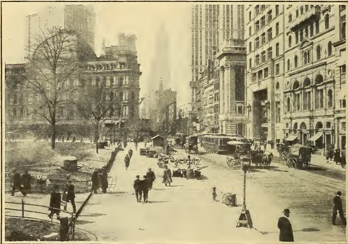
Broadway at City Hall Square Showing How the Street Surface and Sidewalks Have Been Replaced by Heavy Timber
