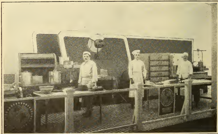
An Electric Grill with a Capacity of 200 Steaks an Hour and an Oven Capable of Baking 160 Loaves of Bread in the Same Period
