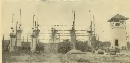
Oil Wells Drilled in the Sea. Their Product is Mixed with Salt Water Which is Extracted by Electrolytic Process
