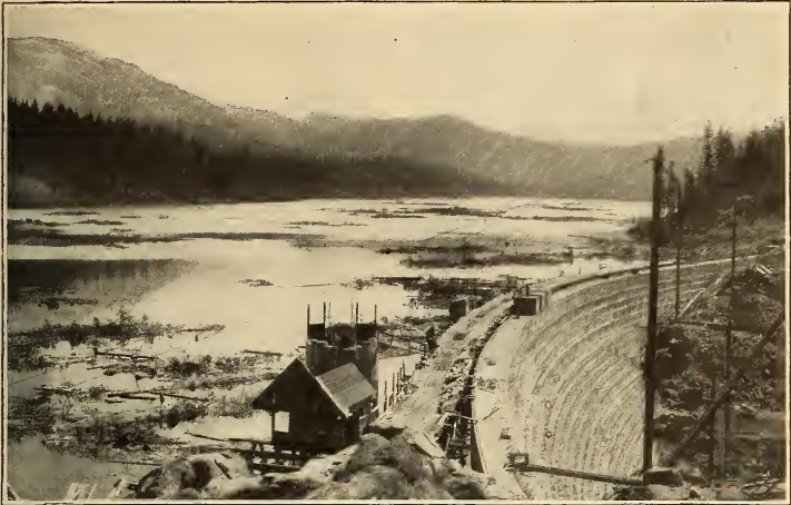
The Mountain Meadow is Now Under Water. Reservoir Near Dam No. 1
