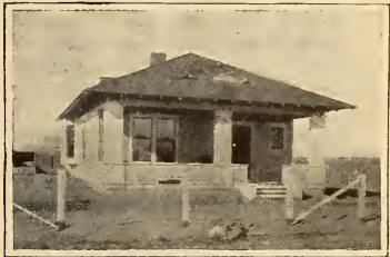
Cozy Bungalow Lighted and Heated by Electricity
