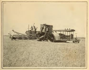
The Harvester is Drawn by a Gasoline Tractor Which Also Carries a Dynamo. The Latter Furnishes Electricity to a Motor on the Harvester for Operating its Complicated Mechanism
