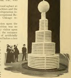
Freezing Temperature of the Pipes Seizes Moisture from the Air to Form a Frost White Fountain attention to an ice machine which it operated and with which a solid mass of ice as big as a good sized story and a half cottage could be made from water in 24 hours.
