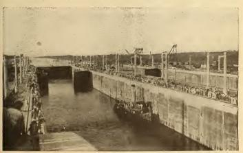
Tugboat "Gatun," first to pass through the locks. It is here shown in the lower lock, with the water up to the center of the lock level and the north gates closed.
