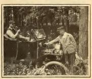
Testing a Telephone Line with an Automobile Magneto
