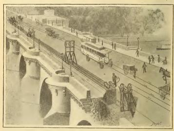
Helicoidal Saw Used in Cutting Through the Pont Neuf in Paris
