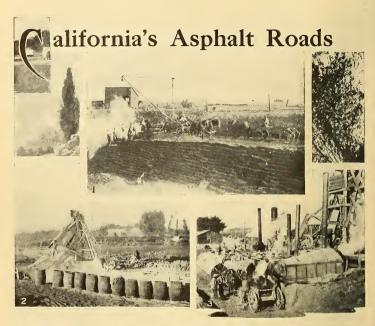
(1) An Asphaltum Mine—the Deposit is Removed with Hot Shovels. (2) Rock Crusher at the Mixing Plant. (3) Loading the Asphalt on Wagons at a Temperature of 300 Degrees
