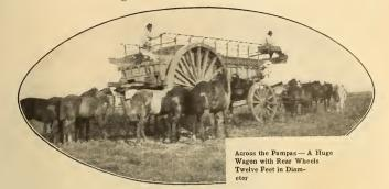
it has farther to sink before the hub is submerged in dust or mud holes, while the greater diameter gives an added leverage in pulling out. An average sized wagon requires eight or ten horses to pull it empty, while with a full load of grain—it will hold almost as much as a flat car—anywhere from 20 to 40 may be used.
