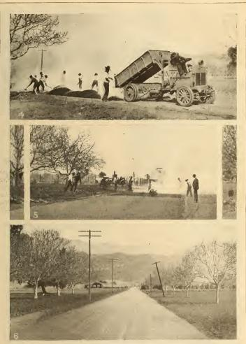
(4) Self Dumping Motor Truck of Five Tons Capacity which Operates at an Expense of 81
