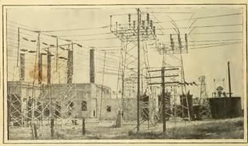
An Outdoor Sub-station in California Where 150,000 Volt Current is Controlled
