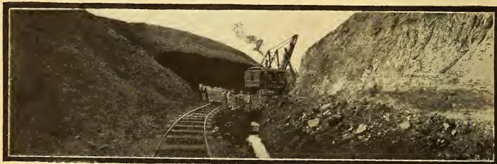
Steam Shovel at Work in a Surface Mine
