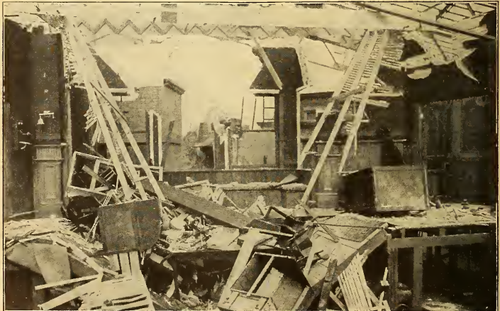
The Aftermath of the Earthquake — All Down in Two Seconds
