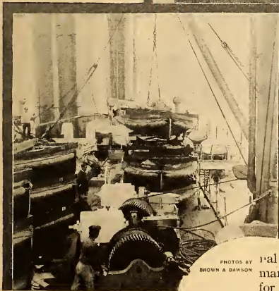
The life boat davits are all of the very newest type as shown at the right. They are operated with winches driven by electric motors as shown in the picture above and each winch is readily controlled by one man.
