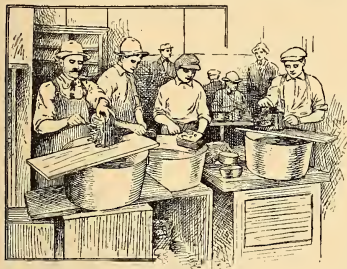
Scrubbing Meter Parts with Toothbrushes
