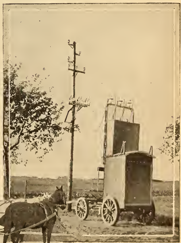
USE OF A PORTABLE TRANSFORMER IN GERMANY FOR SUPPLYING FARM DISTRICTS
