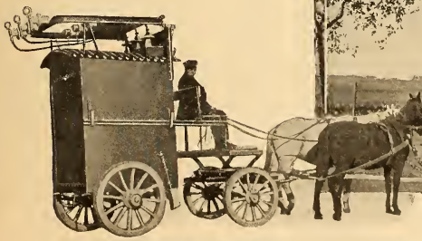
USE OF A PORTABLE TRANSFORMER IN GERMANY FOR SUPPLYING FARM DISTRICTS
