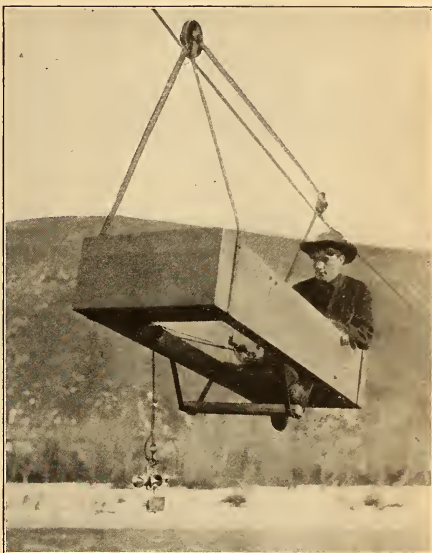
Photographs by Courtesy of Stone & Webster. OPERATING THE CURRENT METER FROM A TRAVELING CAGE
