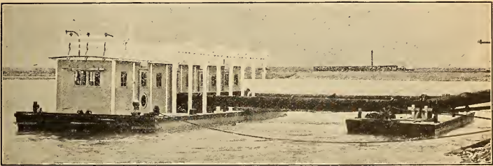
A PUMPING BARGE IN THE MISSOURI
