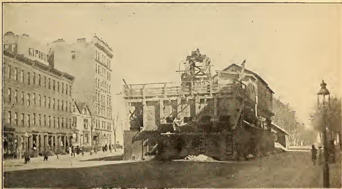
DOWN 200 TO 750 FEET BELOW THESE HEAD HOISTS THE TUNNEL "MINERS" ARE WORKING
