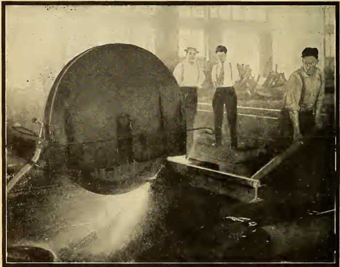
SAWING THROUGH STEEL
