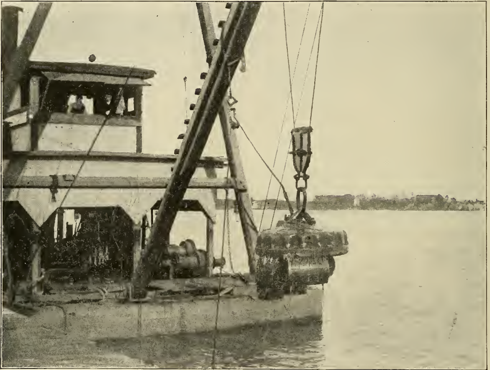
RECOVERING A CARGO OF NAIL KEGS WITH A LIFTING MAGNET
