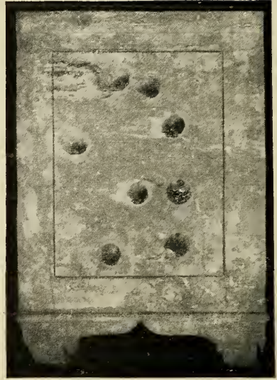
SAFE DOOR PUNCTURED BY ELECTRIC ARC
