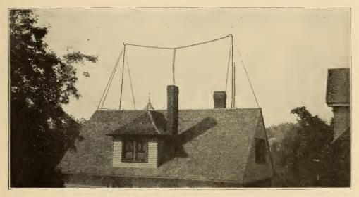
FIG. 22. DOUBLE-ENDED "T" TYPE ANTENNA.
