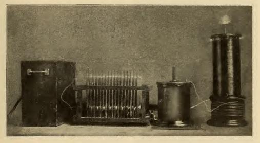
FIG. 1. APPARATUS FOR GENERATING HIGH FREQUENCY CURRENTS.
