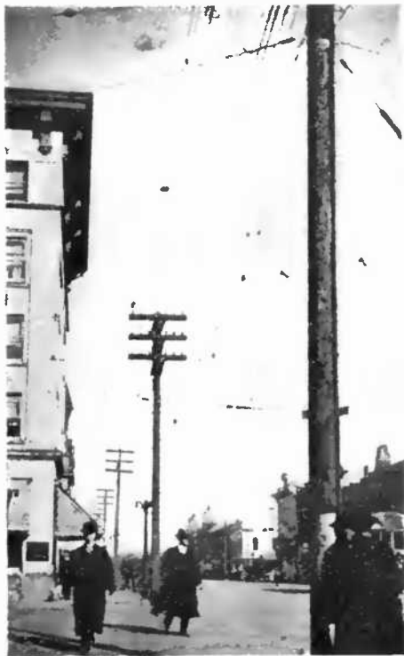
The Old-time Practice of Using Poles for Supporting Overhead Electric Wires.
