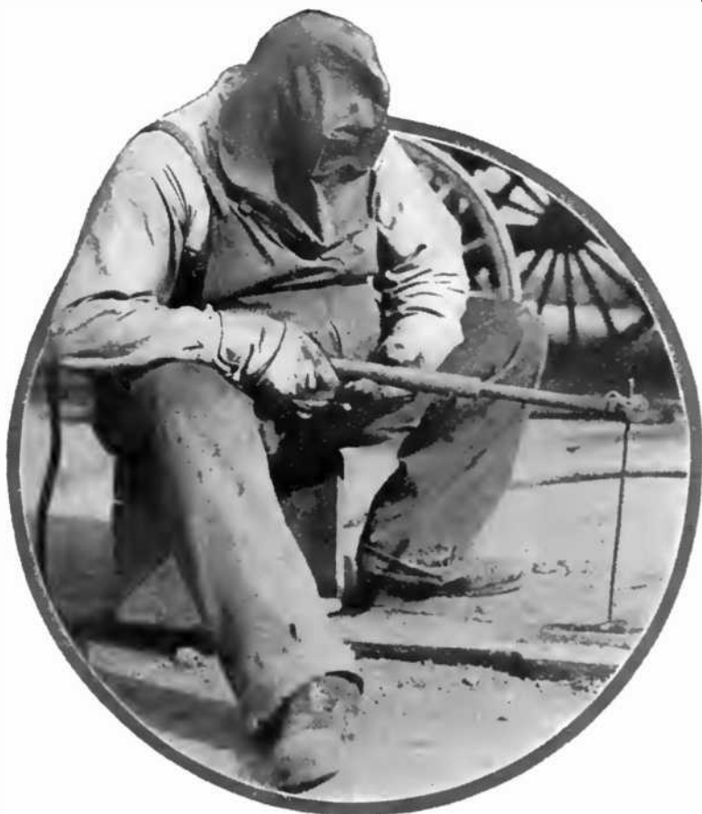
Workman Using an Electric Arc for Welding Street Car Rails.
