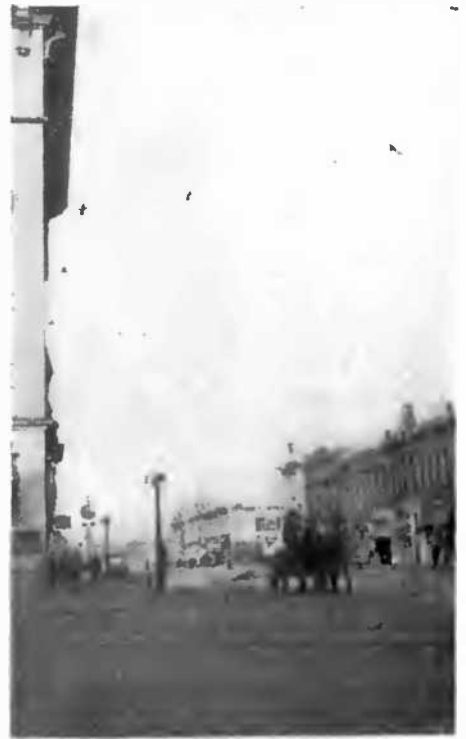
A Modern Street Scene, Showing the Elimination of Poles and Overhead Wires.
