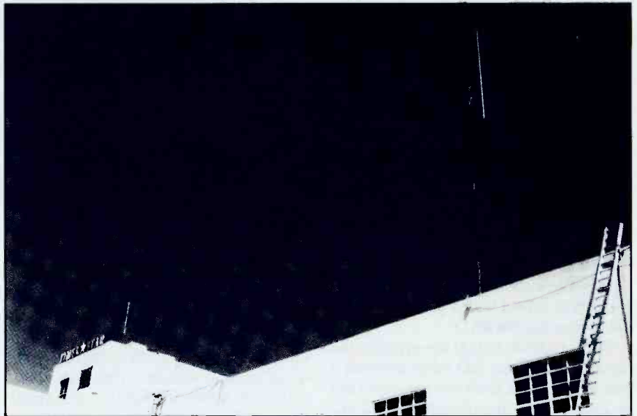
The old KONG-FM tower and five-bay antenna shown at the right in this photo taken last year, nearly half a century after the station went dark! (Photo by Jan Lowry, Castaic, CA).
