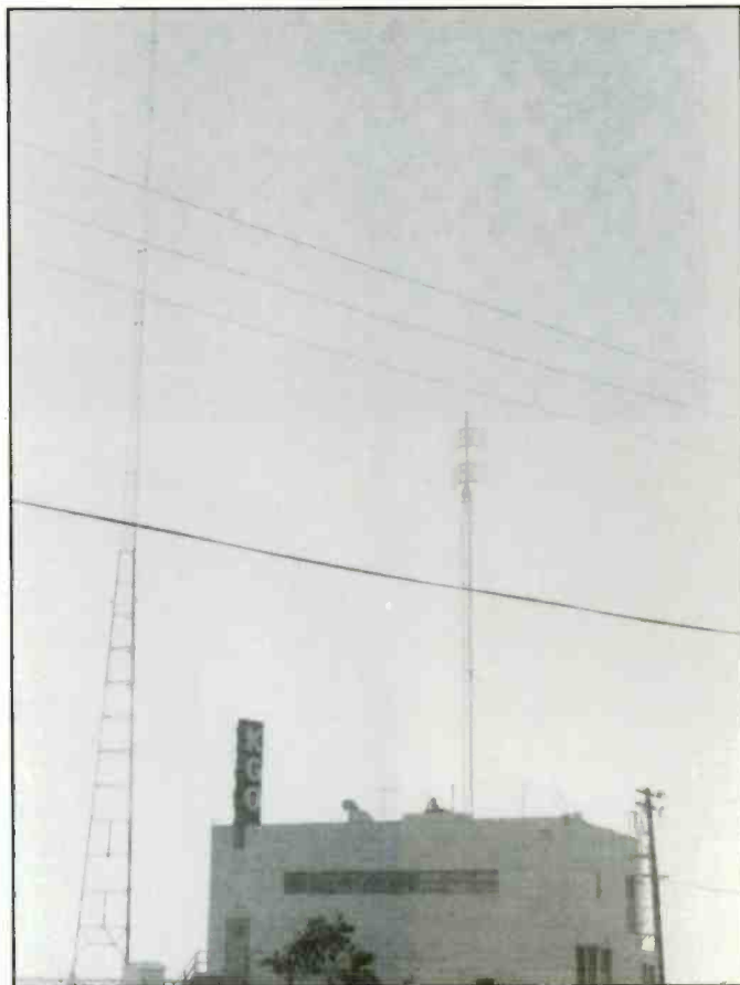
KGO's transmitting plant, as it looked in 1979. (Photo by Jan Lowry of Broadcast Pro-File.)
