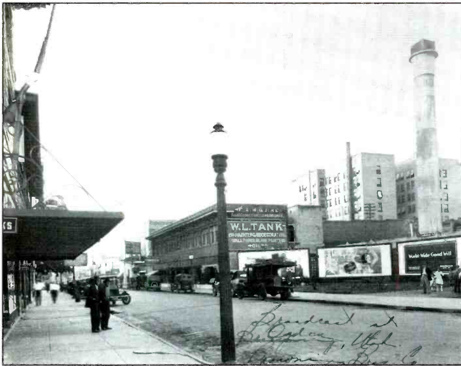
The Zenith mobile radio station, using the call letters WSAX, broadcasting across the street from Browning Bros. Co., Ogden, Utah. (Courtesy Alan Douglas)
