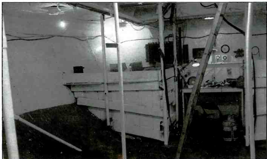
M/V Fury's transmitter room after the FCC visit. Look Ma, no transmitters!
