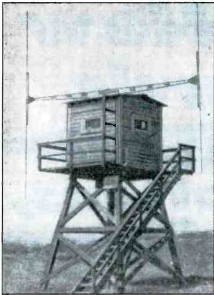
Typical RID secondary monitoring station, showing the Adcock DF antenna. It had to be rotated by hand from inside the shack.
