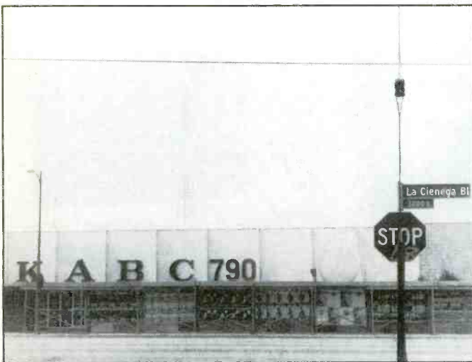
The old KABC building in Los Angeles, built around 1960. Photo taken last March on the day it was torn down to make more parking space for the new KABC/KLOS facility, nearby. (Photo courtesy Broadcast Pro-File, Hollywood, Calif.)
