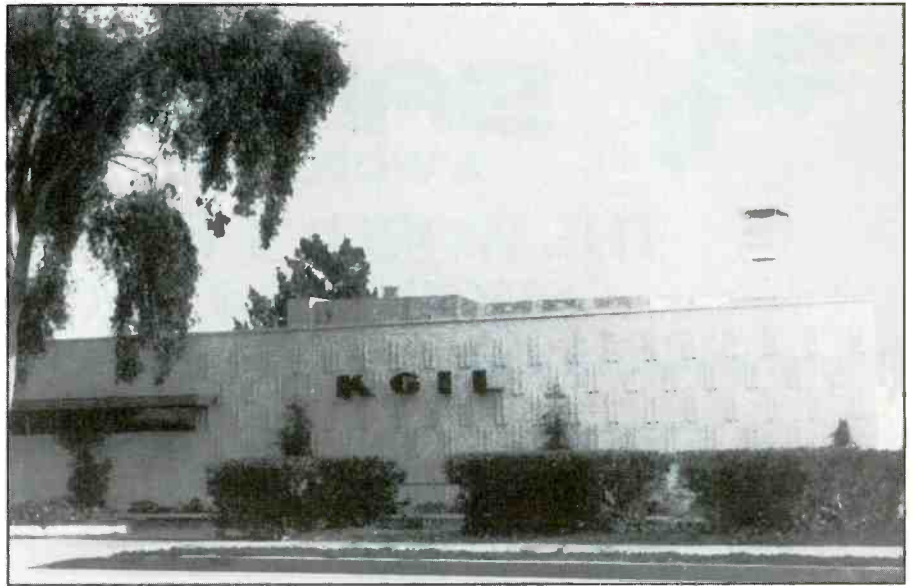
Photo of the KJQI, San Fernando, Calif. (former KGIL) transmitter building, which double as studios for FM'er KMGX, Mission Hills. Photo taken last January. On AM, the station uses the double ID of: "K-Joy AM 540 and 1260." (Photo courtesy Broadcast Pro-File, Hollywood, Calif.)
