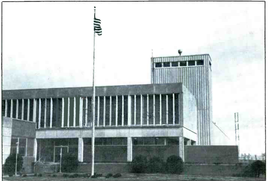
The main building at the VOA Greenville transmitter site. Photo courtesy A. Nunnery, NC.
