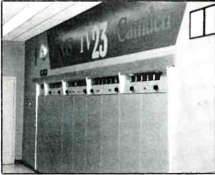
The RCA TTU60B transmitter and associated exciter and driver at UHF-TV station WNJS. (Courtesy Jim Esposito, NJ.)
