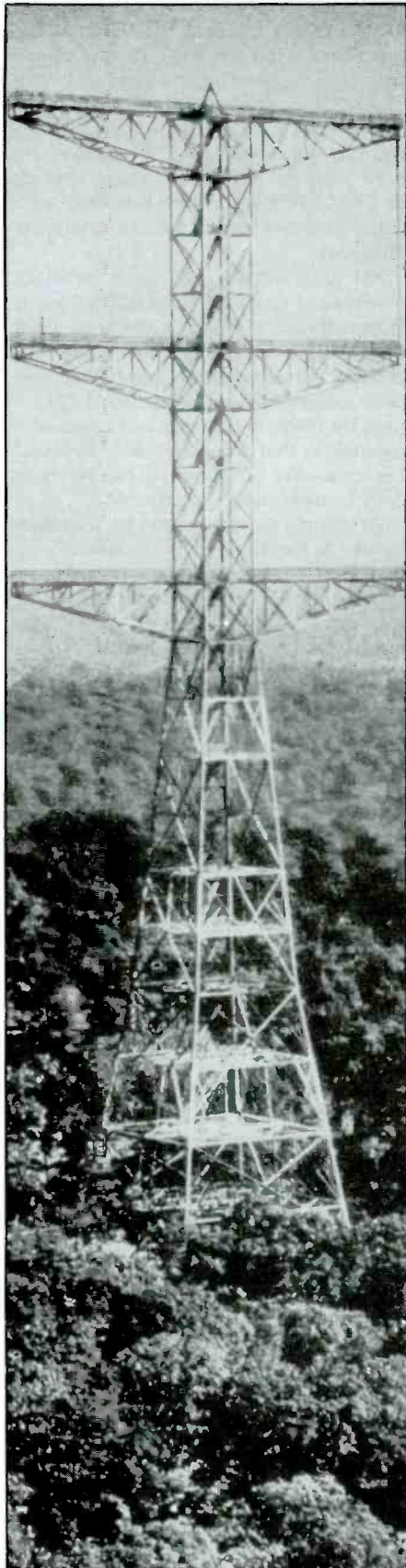
The 400 ft. antenna tower at Alpine, NJ used by Armstrong's station W2XMN. No swivel-chair supervisor, Armstrong dangled in a bo'sun's chair from the crossarms to get the antenna elements tuned to perfection.
