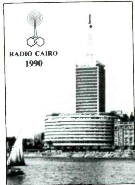
Maybe the same effect which caused this photo of Egyptian Radio and TV headquarters also causes the poor modulation on Radio Cairo!
