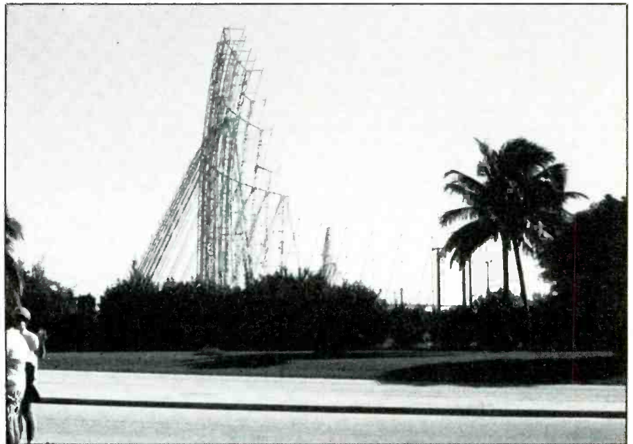
This large array is located at Freeport, in the Bahamas. Local residents told me that it's owned by the U.S. Government and is part of the anti-smuggling efforts based there.
