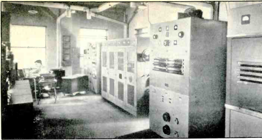
WWZR's transmitter room in late 1943. The rig generated 18 kW, but the antenna gave it a 50 kW punch.
