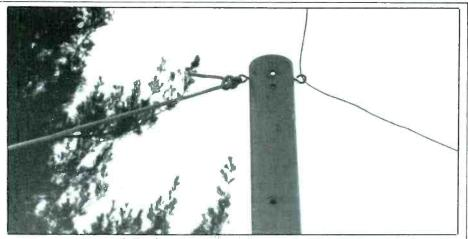
Figure 4: Feeding zig-zag through eye-ring at top of 10' mast.
