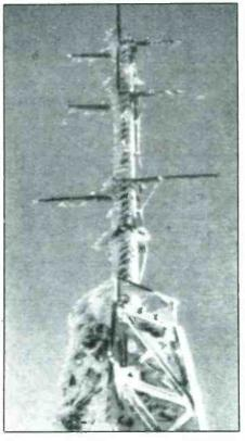
The turnstile FM antenna at W1XER/ W39B atop frozen Mount Washington. It had to have spring-loaded elements to keep them from snapping under the weight of tons of snow and ice.
