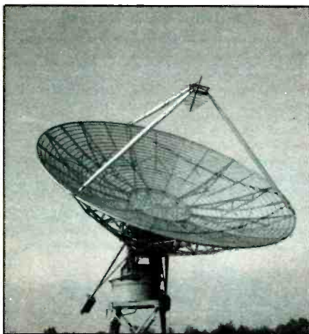
28-foot dish with log-periodic feed for 90 MHz–1300 MHz, circa 1964.
