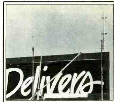
For quick base station communications for security and other operations, base station antennas are attached to this racetrack sign in the infield at Pocono International Raceway in Long Pond, Pennsylvania. (Photo by Chuck Gysi, N2DUP)
