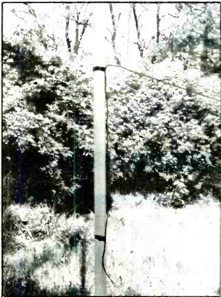
Figure 5: Swing coax line back to mast in a loop away from center feed-point of sloper.
