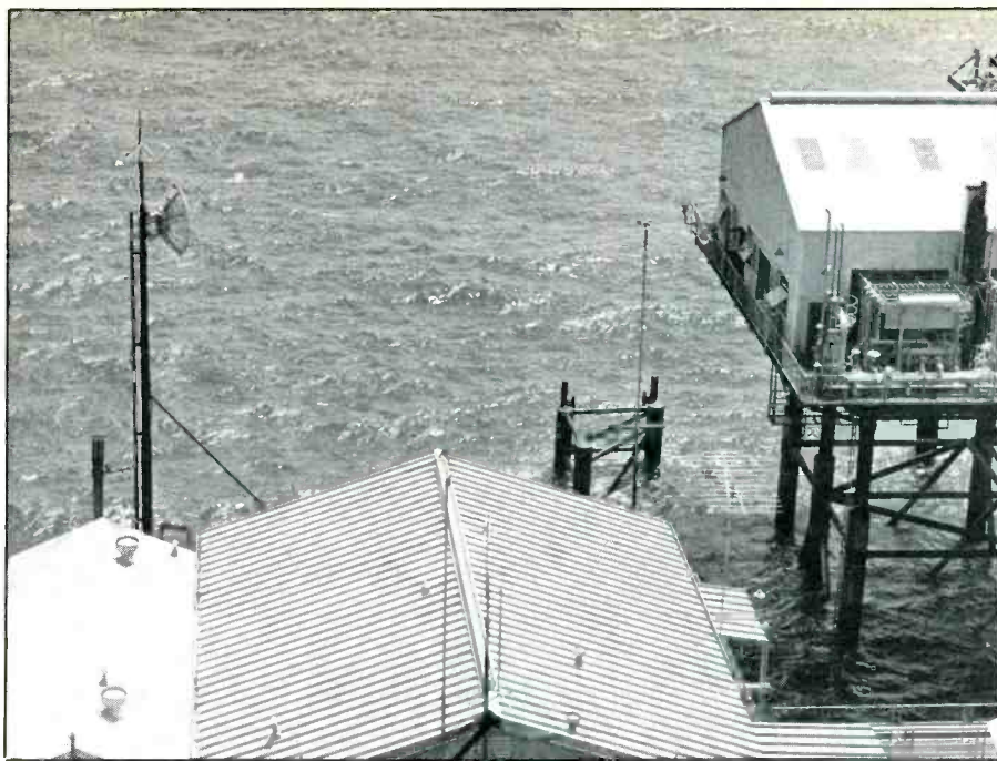
This is a close-up of some of the antennas on a modern off-shore oil rig. (Photo courtesy Mobil Oil)
