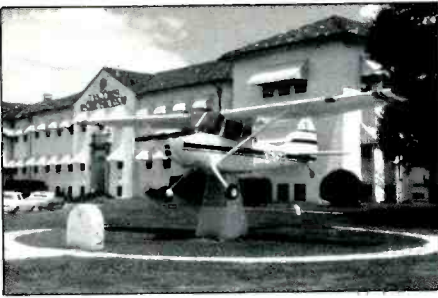
National Headquarters, Civil Air Patrol, located at Maxwell AFB, Alabama. The 0-1 "Bird Dog" aircraft on display in front of the building was dedicated on December 9, 1983, in memory of those CAP members who gave their lives in service to the nation. (Photo by SSgt. Rand McNatt, USAF)
