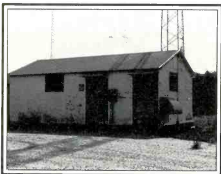
Closeup view of the transmitter building. The paint was peeling but, all in all, it seemed to be in good shape; and all of the transmitting gear could be seen through the windows and looked to be intact.
