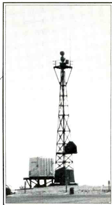
Coast Guard radio beacon "EIN" operates on 311 kHz from Long Island, New York.
