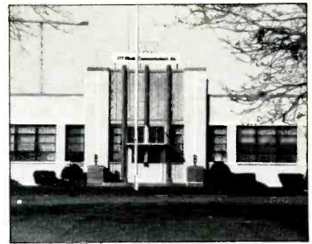
The transmitter building for WSL's short-wave operation.
