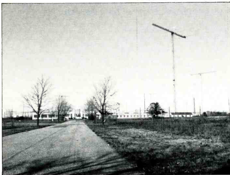
The overall view of the ITT World Communications site at Hauppauge, New York. This is the origin of the WSL signals.
