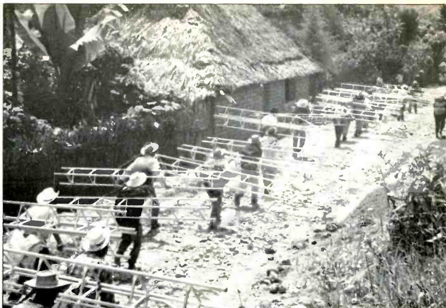
Sections of the antenna tower are carried up the mountain, later to beam the programs of Radio Maya Barillas in Guatemala.
