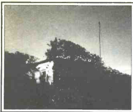
The radio shack weather-worn but still standing on Darby Island.
