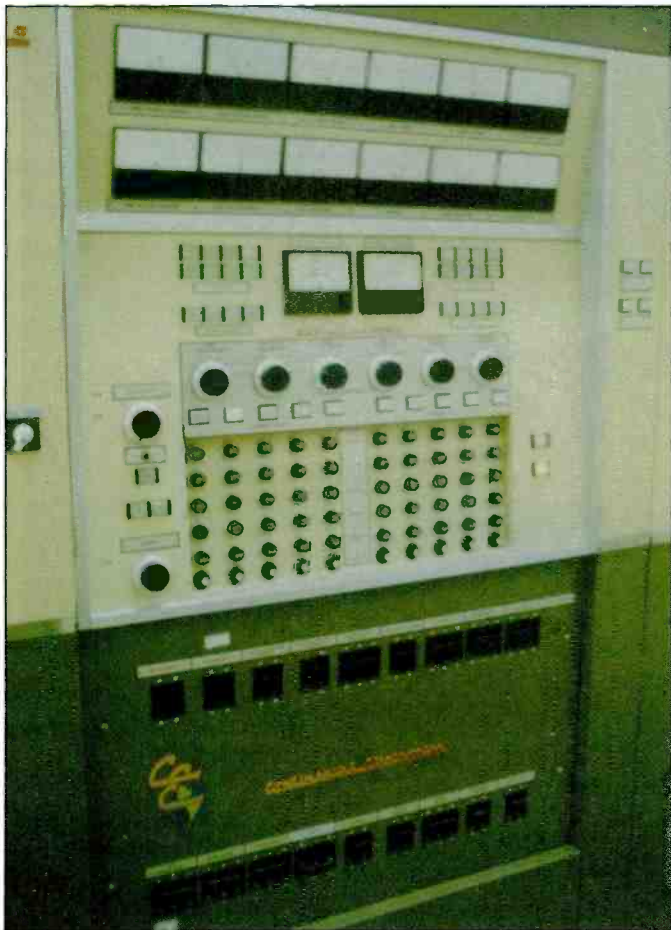
One of the transmitters used by the ABC Northern Territory Shortwave Service.
