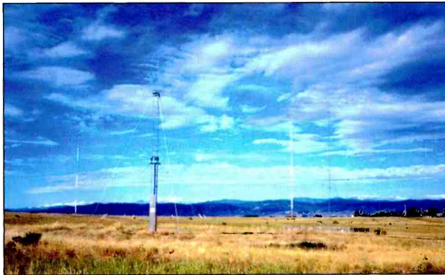
Photo D. WWV, in Fort Collins, Colorado, radiates 10,000 watts on 5, 10 and 15 MHz; and 2,500 watts on 2.5 and 20 MHz. This is the 15-MHz antenna. (Courtesy of Wikimedia Commons)
