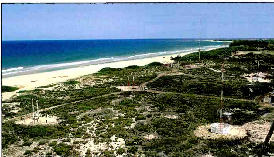
Photo E. WWVH, in Kauai, Hawaii, radiates 10,000 watts on 5, 10 and 15 MHz; and 5,000 watts on 2.5 MHz. (Courtesy of Wikimedia Commons)
