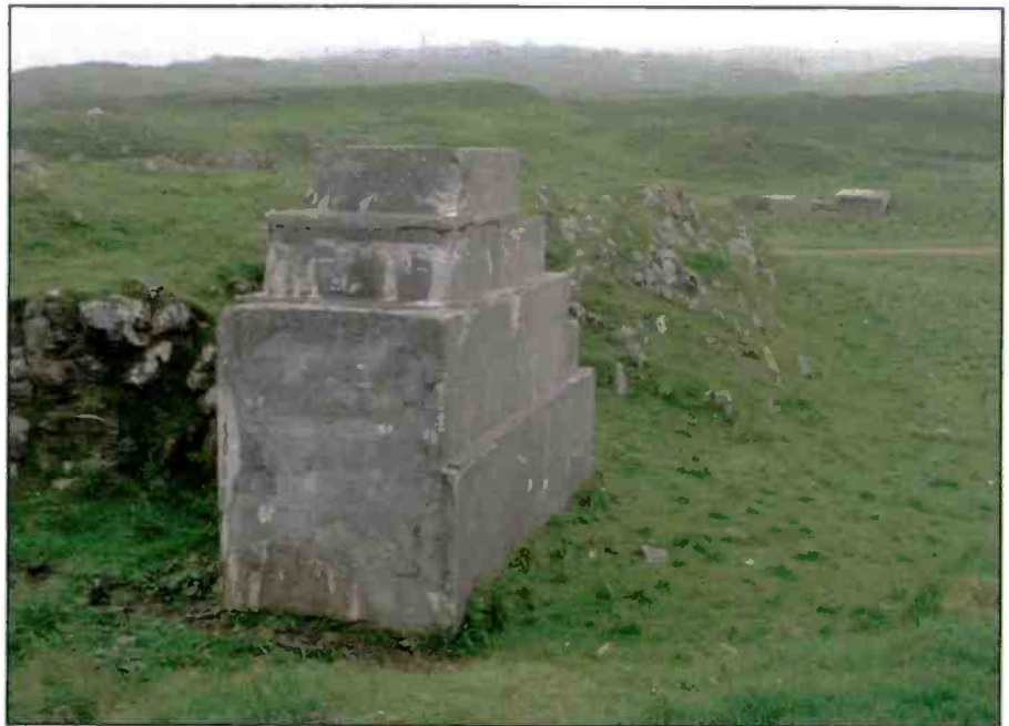
A transmitting station was built here by Reginald Fessenden and in 1906 made the first two-way radio telephony transmissions between here and Brant Rock in Massachusetts from a 450-foot mast. (Photograph and caption by JM Briscoe, courtesy of Wikimedia Commons)
