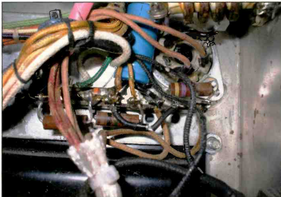
Photo J: The minus 49-volt bias supply after replacing all of the capacitors, out-of-tolerance resistors and the early silicon diode.
