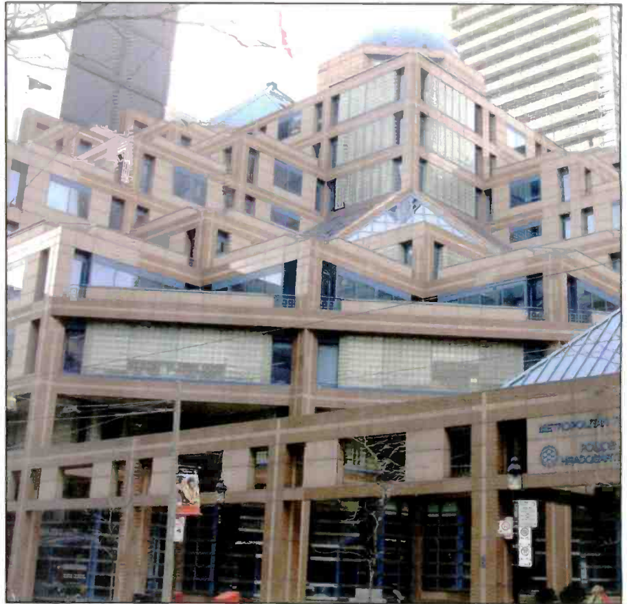
The Toronto Police Headquarters Building in downtown Toronto is an interesting deviation from the typical police headquarters building. (Courtesy of SimonP)
