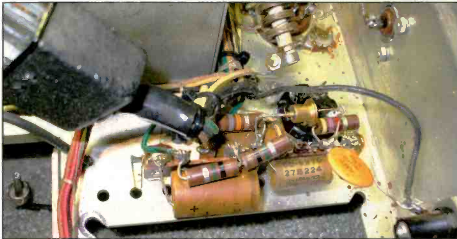
Photo I: The majority of the minus 49-volt bias supply components are mounted on the terminal strip. Note the replacement early-style diode that was used to replace the original selenium rectifier at some time in the past.
