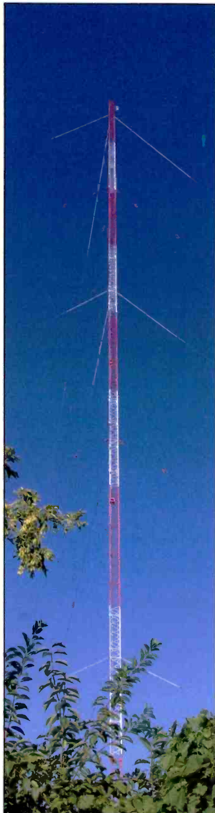
Transmitter tower for sports talk station WSCR-670 in Bloomingdale, Illinois, as seen in July 2010. If you're east of the Rockies, give the station a try. The author heard it in early 2010 in New Mexico.
