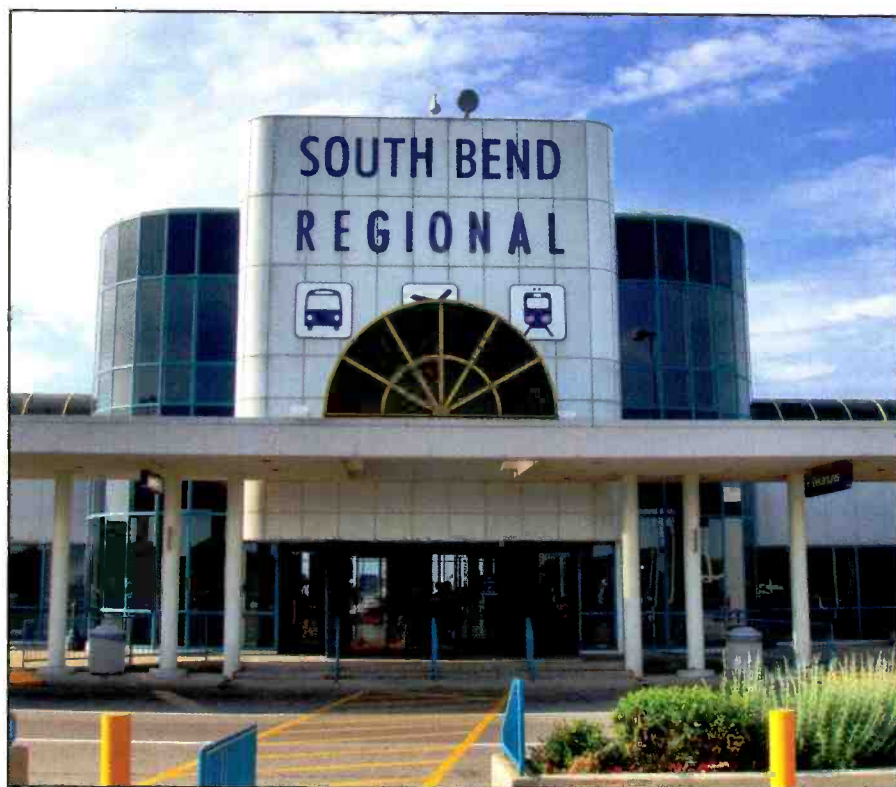
The remodeled terminal at South Bend. (Wikimedia image)
