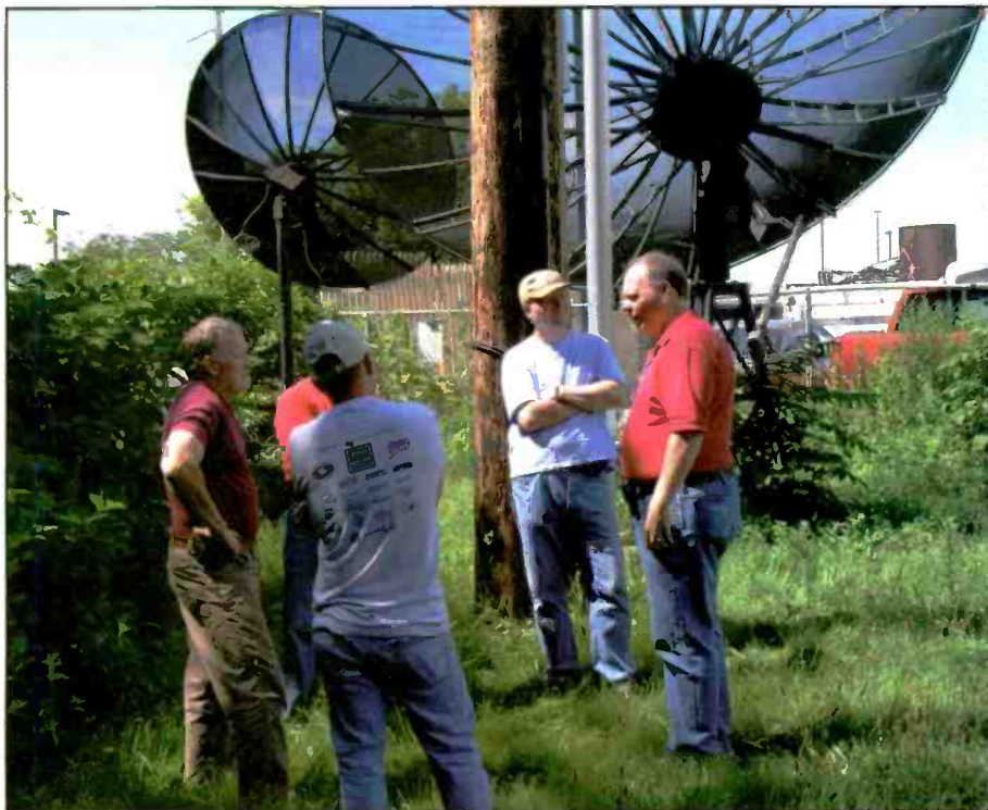
Members of the North Hills Amateur Radio Club and employees of Hollidaysburg, Pennsylvania-based MultiComm, Inc., prepare to put up a new UHF antenna for use by the club's D-STAR repeater. (NHARC photo by Bob Morris, K2RK)
