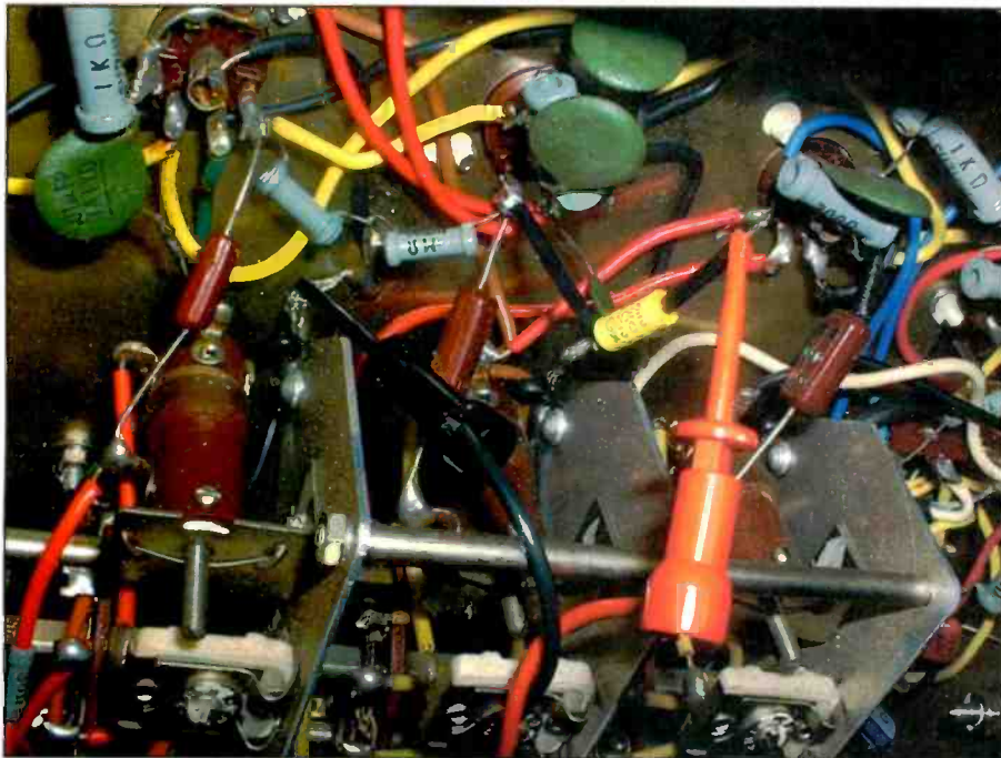
Photo B. A .001 \mu Fd mylar capacitor with a 630 volt rating is connected in series with the output of the center conductor from signal generator's output cable. This protects the generator's precision 50-ohm attenuator from being damaged in case the output is accidentally connected to a voltage source.
