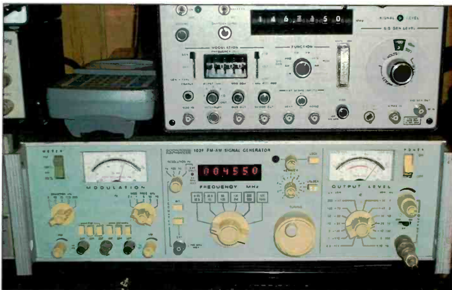
Photo C. The shop's Boonton 102F is set and phase-locked to the HE-10 receiver's IF frequency of 455 kHz. The generator is set for AM modulation, and is modulated with a 400 Hz tone at about 70 percent modulation.
