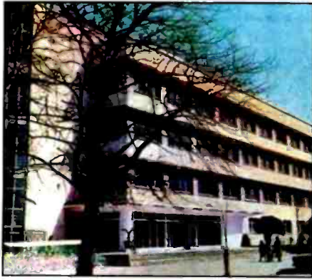
The ARTV Monitoring Center is located here, on the fourth floor of the Radio Tirana headquarters.
