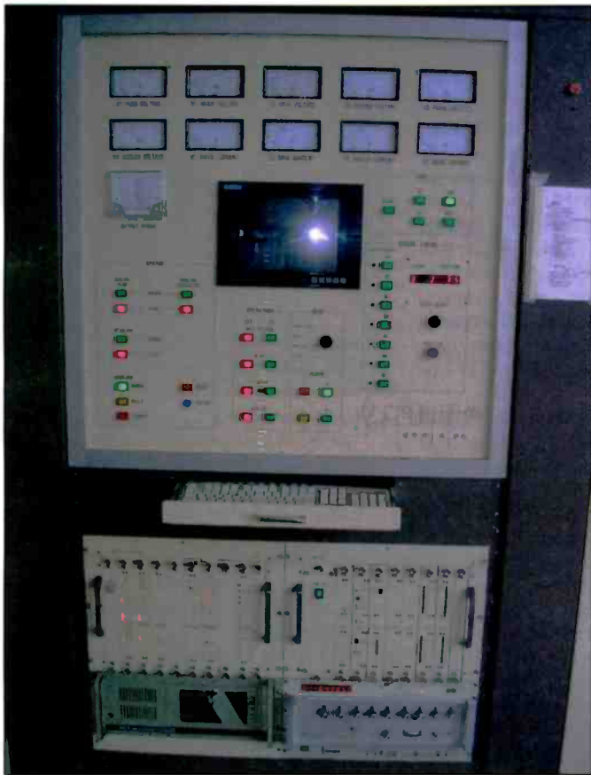
One of the more modern Chinese transmitters, a Continental clone, used for Radio Tirana shortwave broadcasts.
