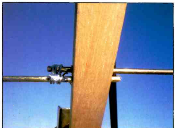
Photo C. Element-to-element connection.
