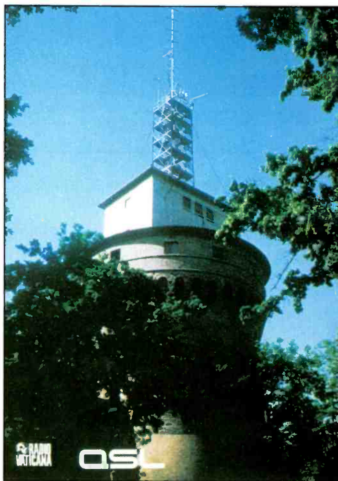
This Vatican Radio QSL shows the antenna for the link between the studio and Vatican Radio's transmitter at Santa Maria da Galeria.
