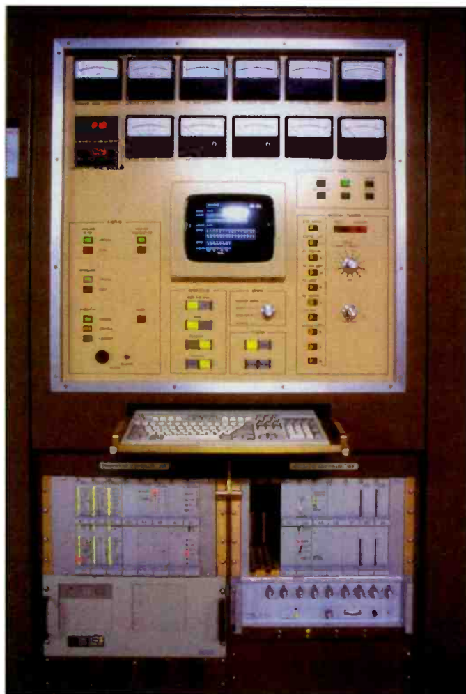
This is what a monster 500-kW transmitter looks like up close and personal. This one belongs to WEWN, Vandiver, Alabama. (Thanks to Charles Maxant, WV)
