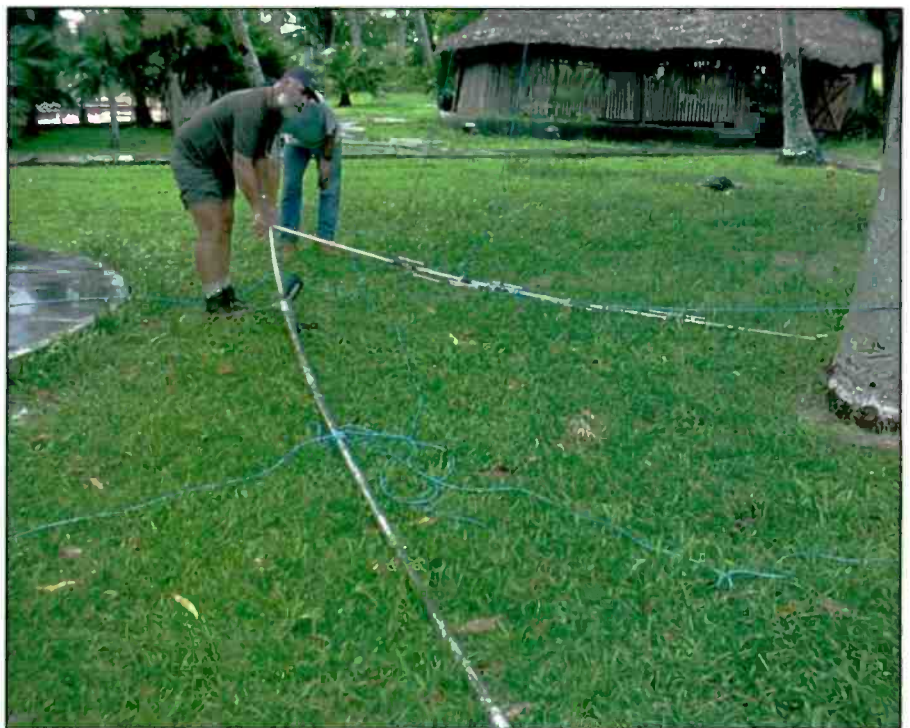
Jorge Novoa, CO2II, inspects damage to a vertical antenna after a windstorm hit the COØUS operating location in Cuba (2003). (Photo by Chip Margelli, K7JA)
