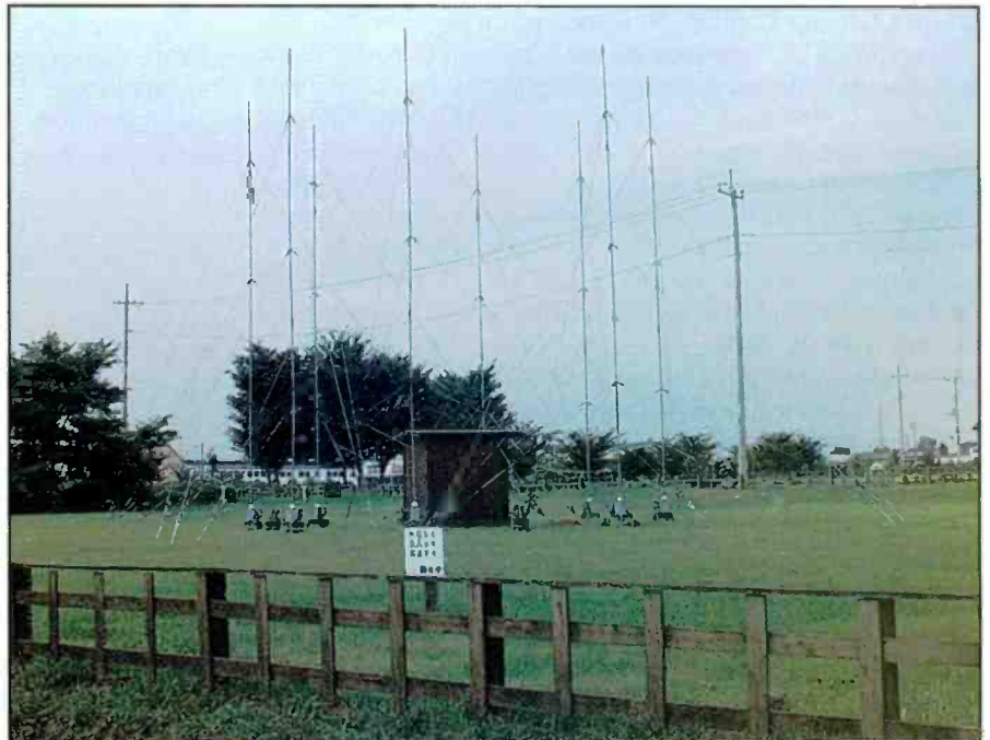
A circular antenna at the Oi station.
