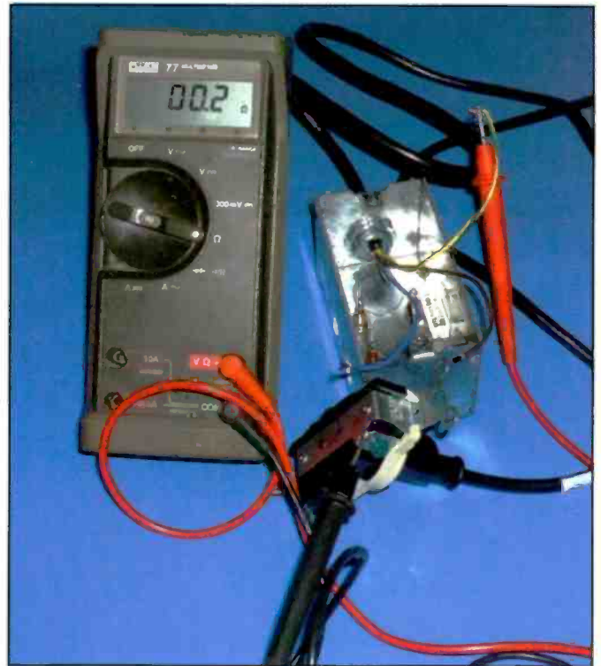
Photo C. The power cord wiring color code did not follow the expected white=neutral, black=hot, green=ground convention. Here, an ohmmeter is being used to verify, and double check, what each lead on the cord is used for.
