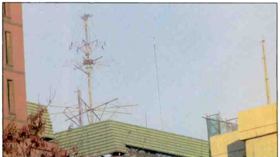
Conical monopole and dipole antennas stand on the top of a Defense Agency building where the Defense Intelligence Headquarters is located.
